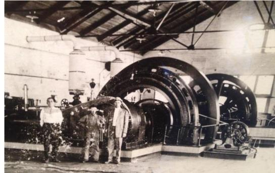
In 1918, a 500 Kw General Electric unit was installed and was served as the main generating unit until 1923. It operated as a stand-by unit until 1949, and was removed from the plant in 1957.
