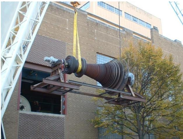
A turbine overspeed incident damaged the 12,500 Kw unit in 2006 causing significant damage. The unit was out of service for well over a year as it was being rebuilt off site. It was redesigned during the rebuild for efficiency.
